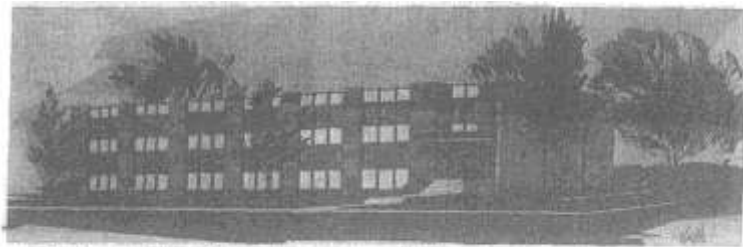
CONSTRUCTION WILL BEGIN in early January, weather per-mitting, on this three-story office building. Located at the corner of Cheno-weth and Dixie, it will be built by the St. Matthews Co., exalters. Based in the building will be the St. Matthews Co., as well as other businesses which will lease space according to their needs. The building will have elevator service.
