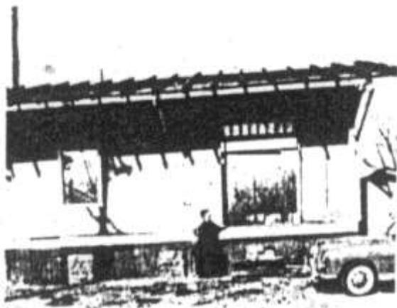
GONE: The old L. & N. train station on Westport Road in St. Matthews is now just a memory. A railroad superintendent is shown examining it last week as it was being torn down. The station, built in 1889, was a landmark. At one time two passenger trains, from Louisville to Lexington, stopped there.
